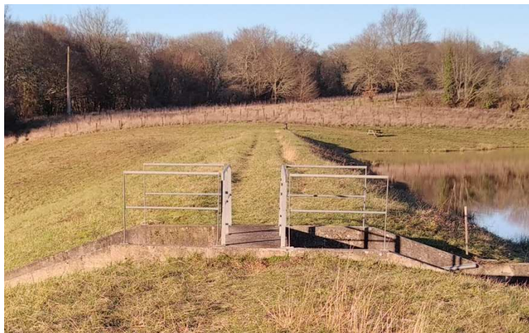
Figure 35 : Barrières garde-corps non conformes
