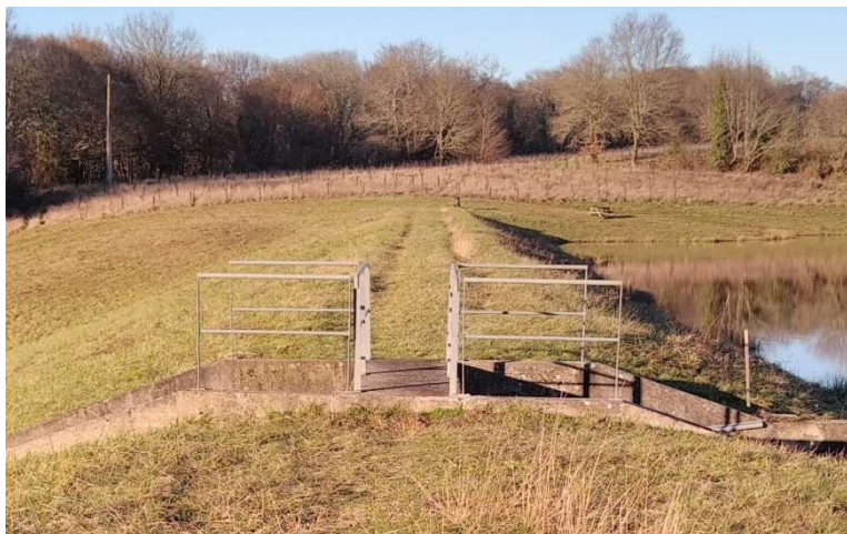
Figure 14 : Barrières garde-corps non conformes
