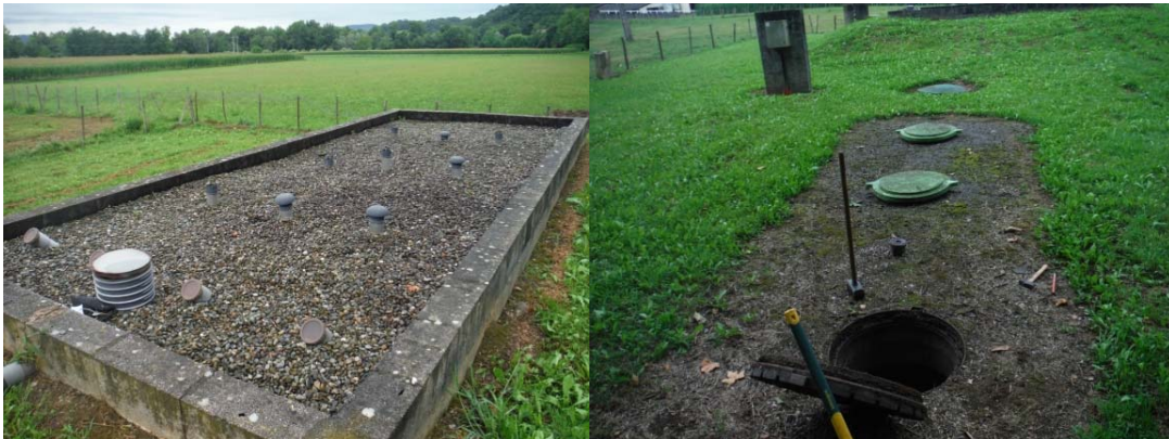
Figure 2 Illustrations de la station d'épuration
